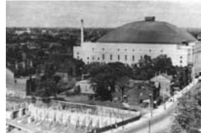
View of Maple Leaf Gardens taken shortly after its construction in 1931, showing the giant domed truss roof that spans the entire interior.
