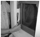
To retrieve the weights for the bottom sash, you will generally find a weight pocket cover in the track that the outer sash slides in. This is approximately 10" up from the sill and held in place with a screw. Many coats of paint may obscure this screw, but it is still there. This cover, which will be about 1 1/2" wide by 12" long, will pull out at the bottom and slide downward, revealing the weights for the bottom sash.
