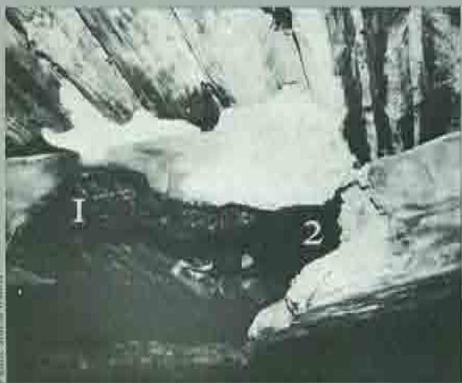
This massive beam snapped dramatically because the wood was desiccated not because it was burned.
