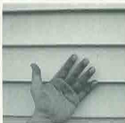
Vinyl siding showing fake wood grain & impact damage (l), and vinyl siding "chalking" (r), evidence of surface breakdown and possibly of siding breakdown.
