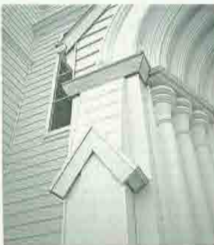
A mid-19th century church in Sackville, N.B. has been clad in vinyl siding, covering fine mouldings and destroying the original architectural character.
