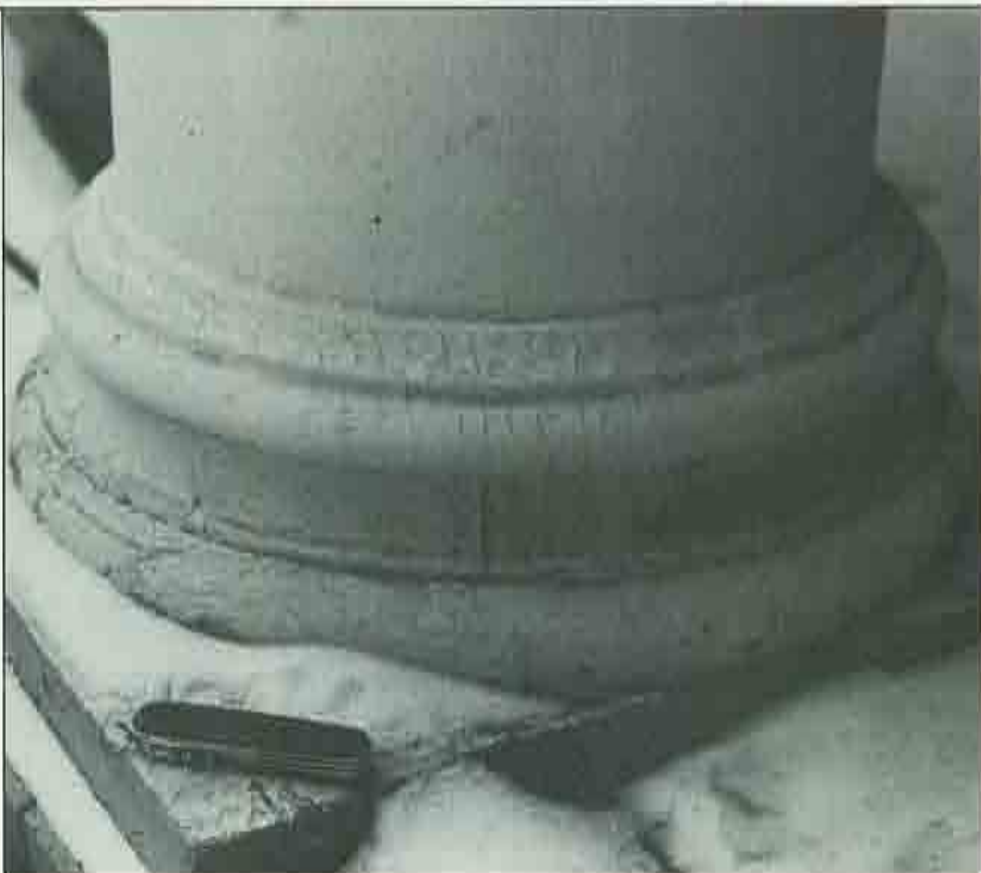
The base of this wooden column shows a combination of cracking and alligatoring. There are so many layers of paint on the mouldings that their profiles are beginning to be lost.
