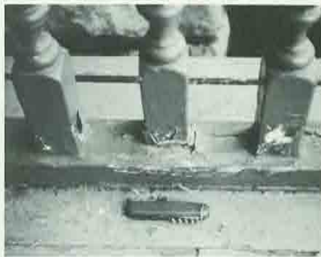
This paint and wood deterioration was caused by snow shovels cutting into protective paint layer.
