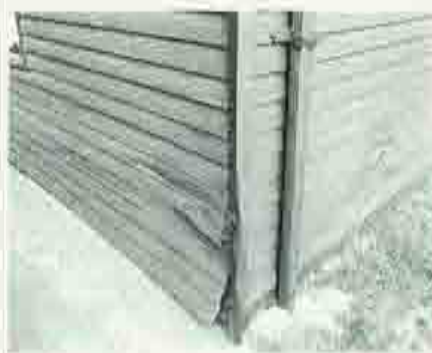
Repainted aluminum siding shows a streaky appearance and is peeling where dented. Also evidence of warping in siding.
