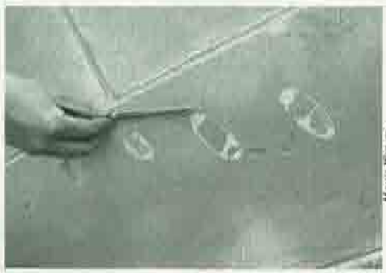
Sulphuric acid in rain eats away marble in Halifax and limestone in Ottawa, where projecting resin provides clue.
