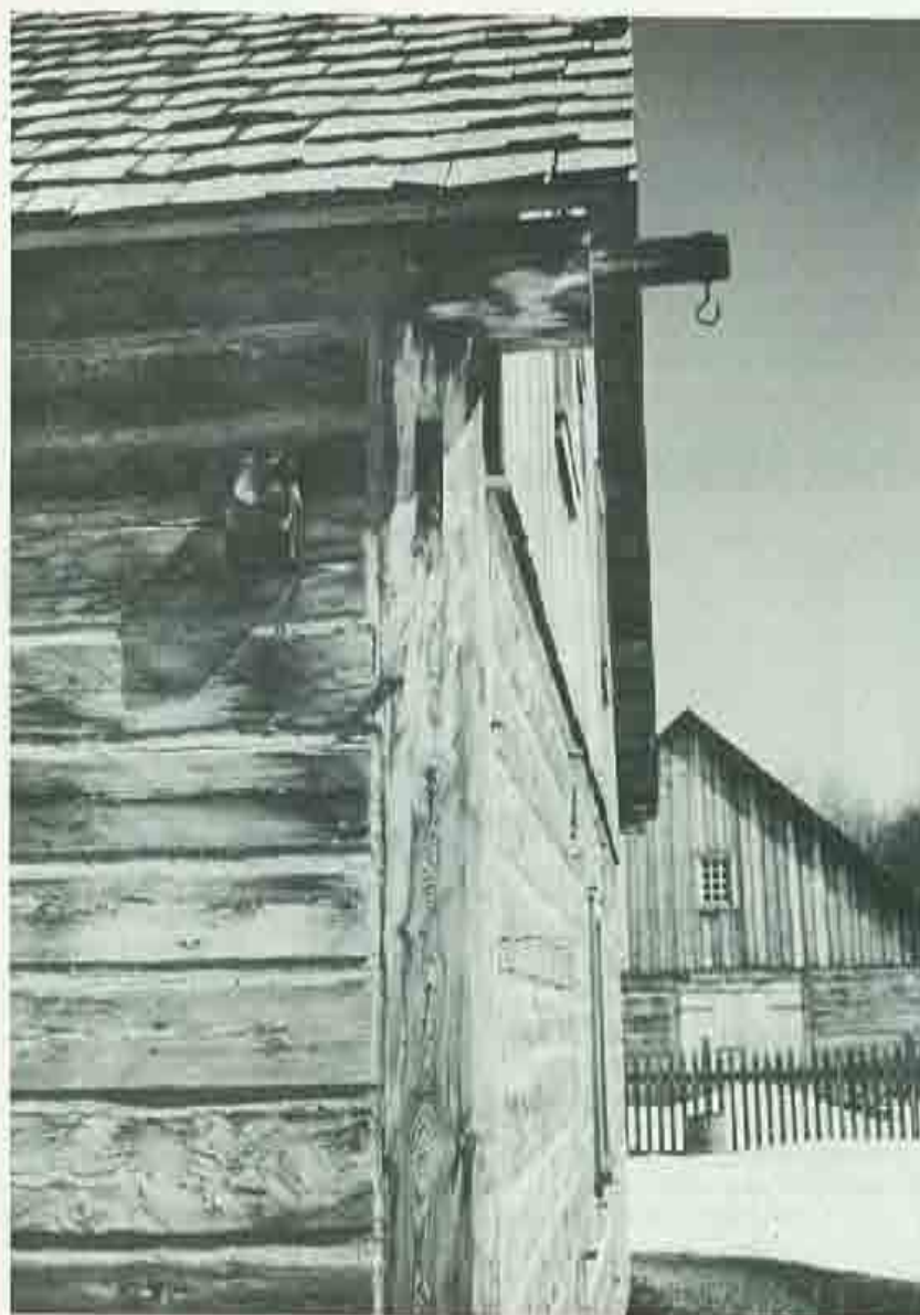
An incorrect application resulted in the whitish green crystalline deposits on the surface of these timbers. The crystals are a lethal mixture of copper, chrome and arsenic salts (a). Such preservative compounds must be properly applied with the correct combination of controlled heat and pressure.
