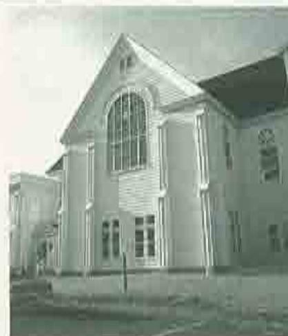
A mid-19th century church in Sackville, N.B. has been clad in vinyl siding, covering fine mouldings and destroying the original architectural character.
