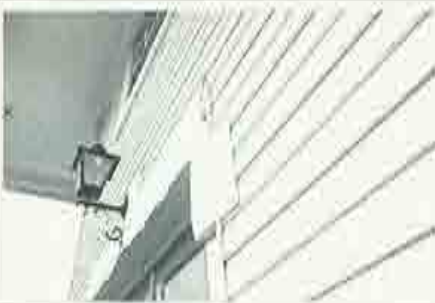
Applying synthetic siding over original siding (left) causes problems around trim. (Right) Painting over deteriorated metal siding: like painting a car with a brush.
