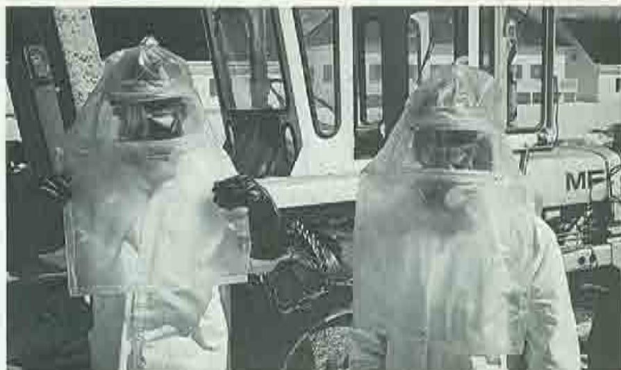
Operatives wearing full protective clothing to apply orthophenylphenol and methanol as a fungicidal treatment.
