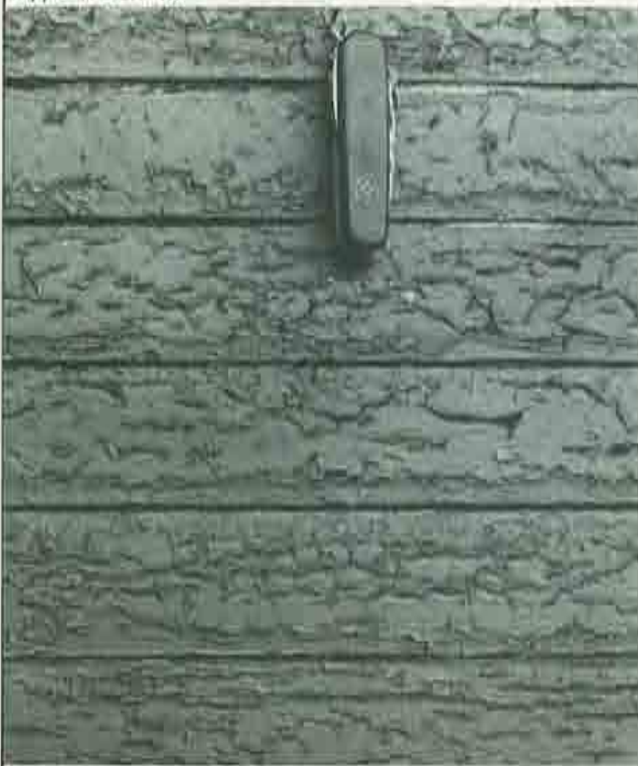
Cracking is here occurring in the heavily painted boards of an old porch deck.
