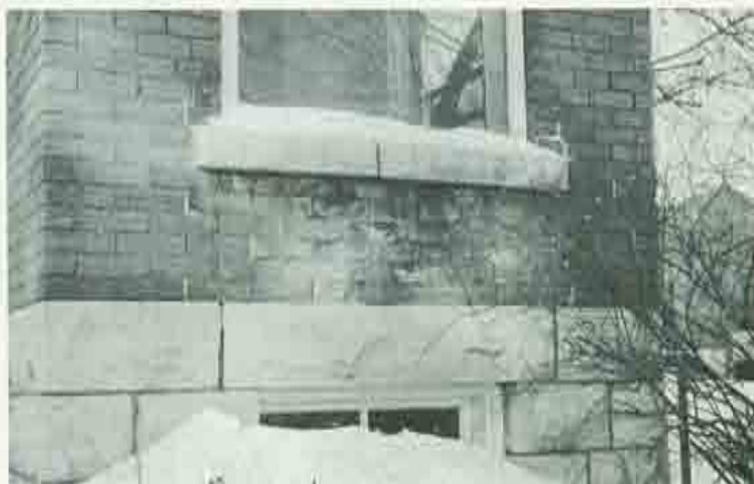
Cracked stone window sills are a common cause of damaging moisture penetration into masonry beneath.
