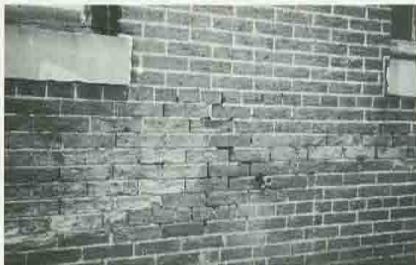
Damp marks and whitish crystalline efflorescence are clues to the cause of the brickwork disintegration.
