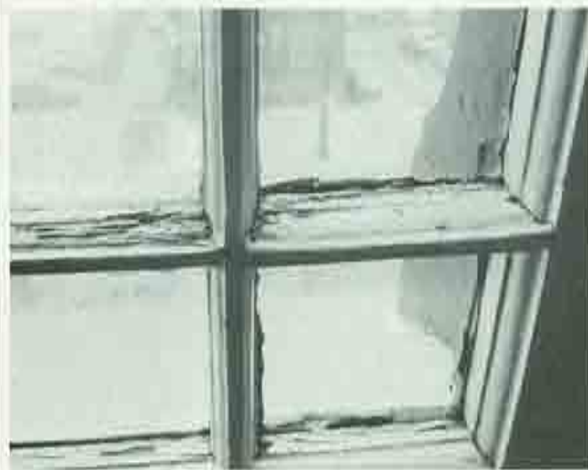
If you get heavy condensation on your windows watch out for paint and wood deterioration.
