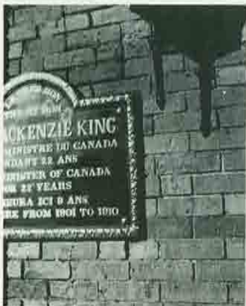
Above left: these bricks and the mortar pointing are part of an historic residence. They show the typical bad effects of an inappropriate sandblasting job. Above right: at the side of the building shown in Fig. 1, one can see the paint which the sandblasting has removed from the front.
