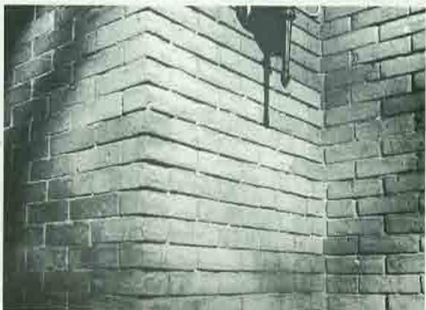
Above left: these bricks and the mortar pointing are part of an historic residence. They show the typical bad effects of an inappropriate sandblasting job. Above right: at the side of the building shown in Fig. 1, one can see the paint which the sandblasting has removed from the front.
