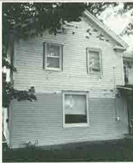
Paint peeling from wooden siding is caused by moisture from building interior—covering it only hides the problem.
