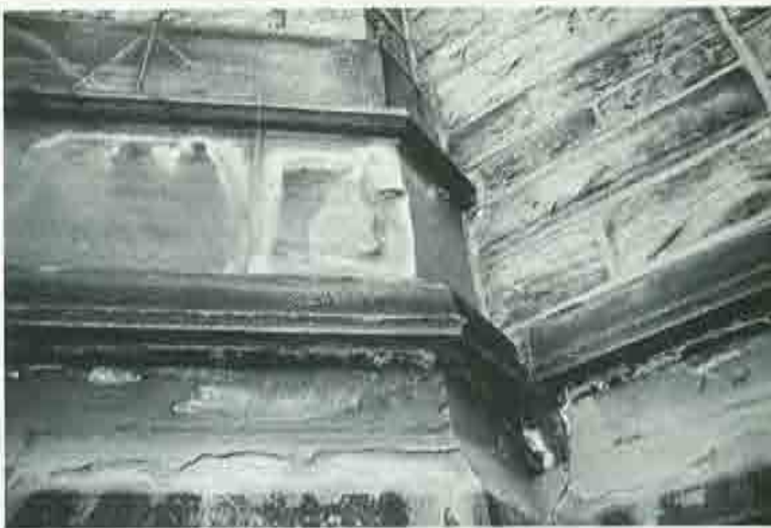
Peeling crusts of sulphate and stone show under a moulding on the right of this detail on the Peace Tower, Parliament Hill, Ottawa.
