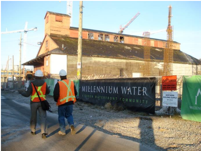
Monitor roof, with a clerestory containing a row of 15-pane windows and cedar ventilation louvres
