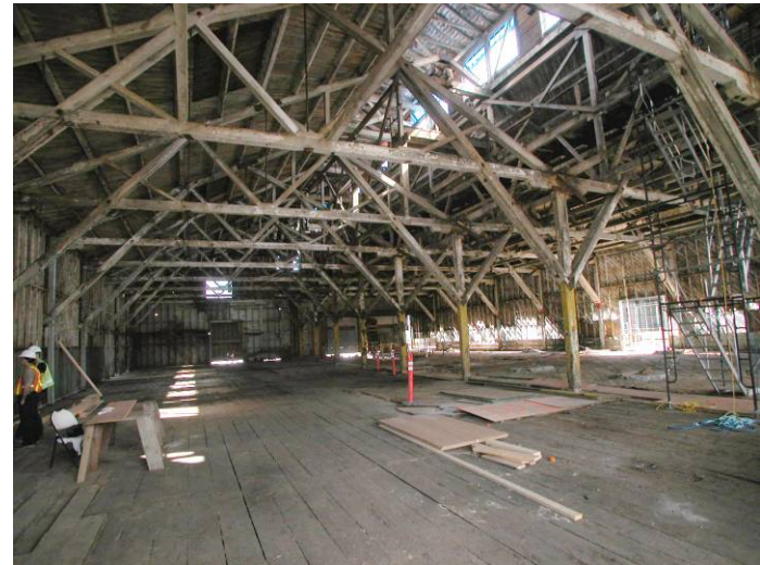
Large, open interior space, interrupted only by a row of columns down the centre
