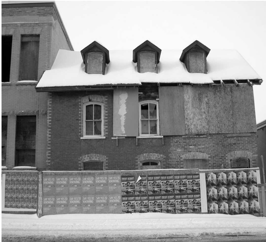
SOUTH FACADE, JANUARY 2009. (M.S.)
