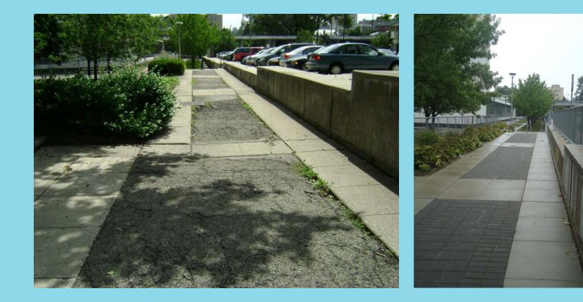
The Building Code and accessibility standards require protection on walls over 600 mm.
