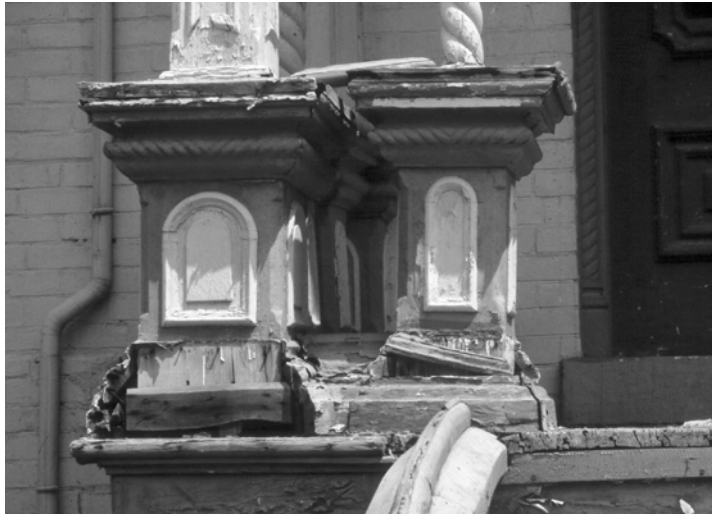
Another example of deterioration beyond rational repair...
