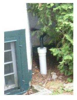
•In 2007 a new sump pump installed due to ongoing basement flooding, no flooding since, but still concern for dampness and potential water infiltration
