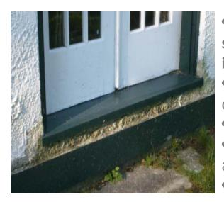
•2009 replacement of deteriorated exterior stucco at sunroom area of museum due to moisture infiltration
