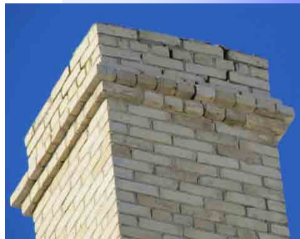
Fig. 28—Loose masonry at the Assumption Catholic Church in Holdfast.
