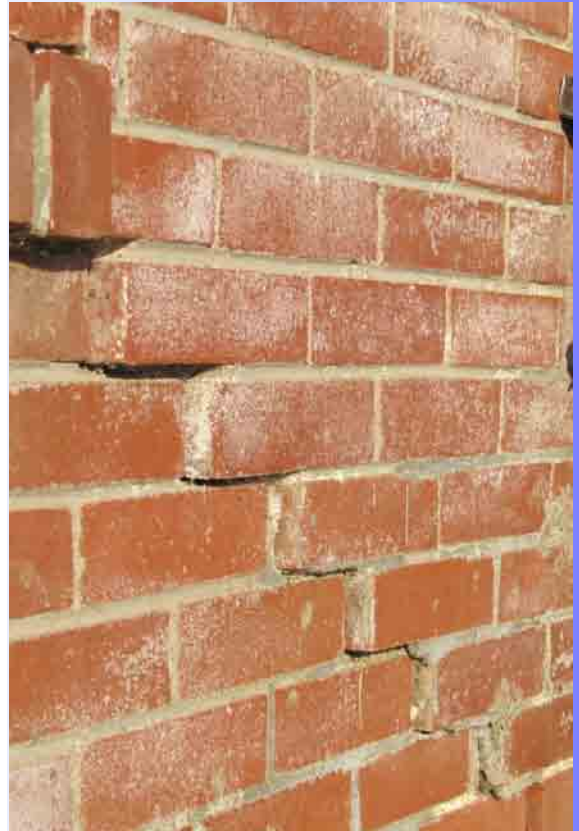
Fig. 13—A masonry wall shifts out of plane at the Veteran’s Memorial Hall in Earl Grey.
