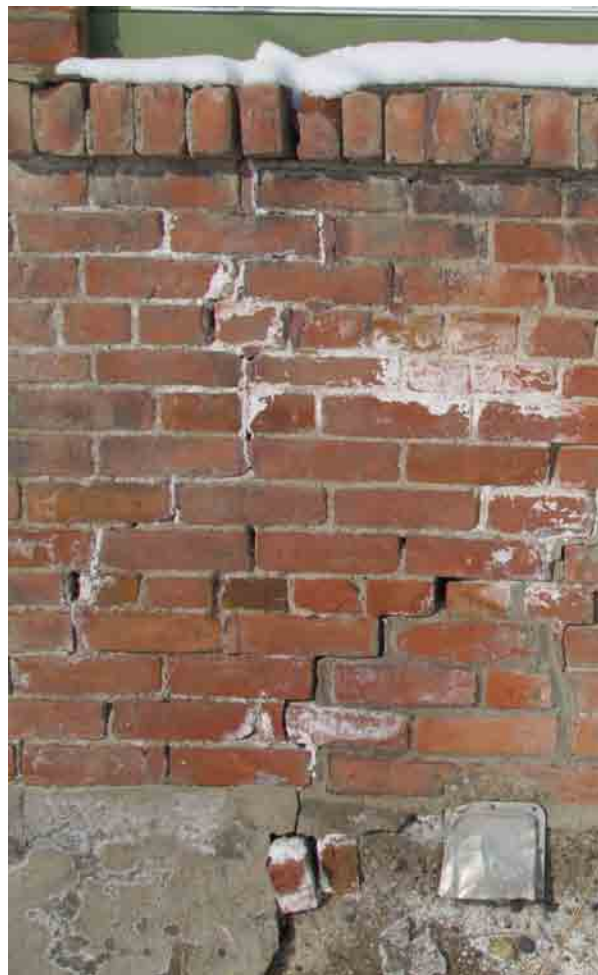
Fig. 15— Soiling and efflorescence at The Stoop, Rouleau
