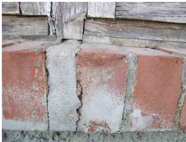
Fig. 19—Mortar joints at the Veteran's Memorial Hall in Earl Grey.
