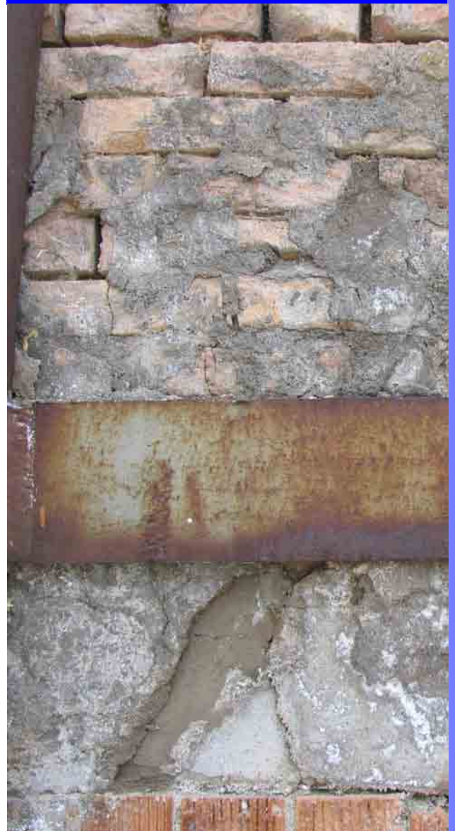
Fig. 18—Previous masonry repairs at a kiln at the Claybank Brickplant, National Historic Site.
