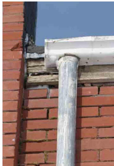
Fig. 6—Masonry damage at a common point of failure at the Khedive Recreation Centre, Khedive.
