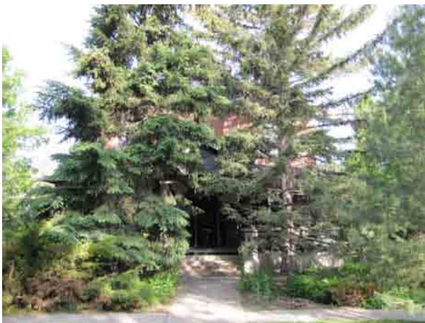
Fig. 12—Residence in Maple Creek showing trees close to the foundation.
