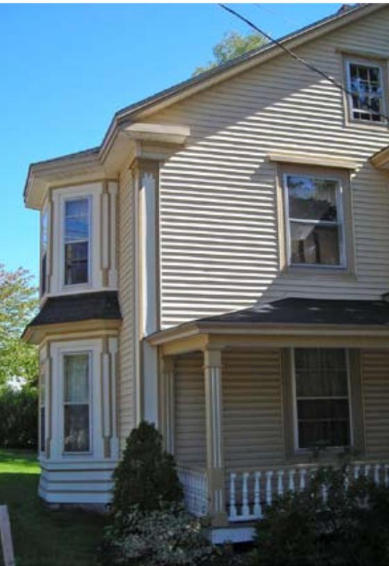
Vinyl siding has been applied to the wall surfaces of this building, leaving the corner pilasters and window trim exposed. The pilasters have become shallower and the windows are now recessed.
