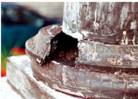
The combination of an impervious metal cladding and failed caulking joints has kept the ongoing decay process out of sight and mind.
