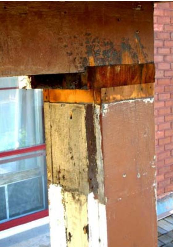
When aluminium cladding was installed on this porch some 20 years ago, several components of this column, including its taper, were removed to accommodate cladding.
