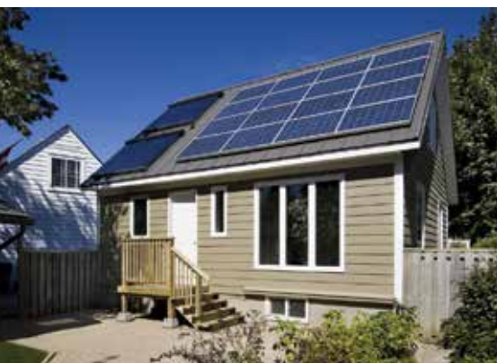
This Now House demonstration project (front and rear views) retrofitted a Victory house in Toronto's Topham Park, reducing greenhouse gas emissions by 5.4 tonnes and electricity use by 60%, while enabling the house to produce enough energy to pay its own bills.
