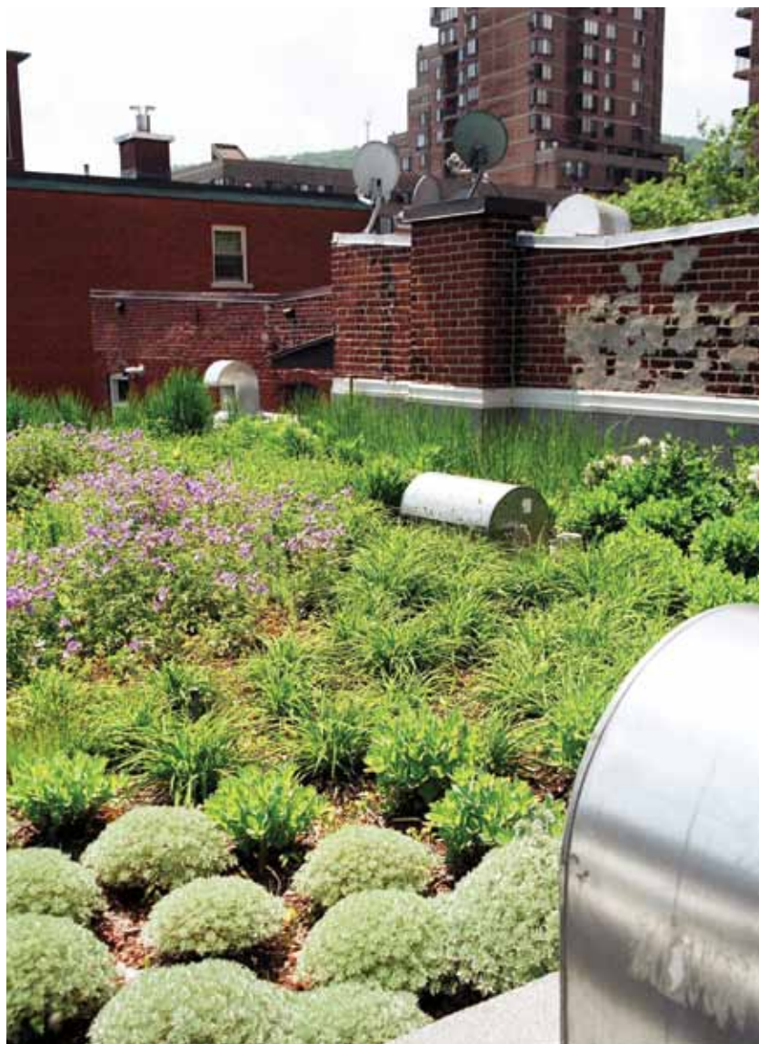
The experimental green roof in Milton Park is divided into three sections: conventional roof, dry green roof and irrigated green roof.
