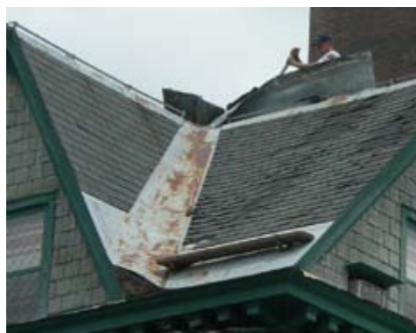
The roof shingles and valley flashing were clearly at the end of their service life.
