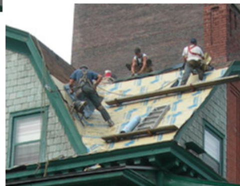
The unusual three-sided valley configuration, which survives from the building's earliest days, was retained and flashed with new metal.
