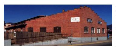
As well as critical upgrades to improve the seismic, electrical and mechanical performance of the building, structural work involved the repair of exterior brick walls and timber roof framing that saw the restoration of the original roof configuration. The project also relocated loading docks and reorganized interior spaces to better meet exhibition space requirements.
