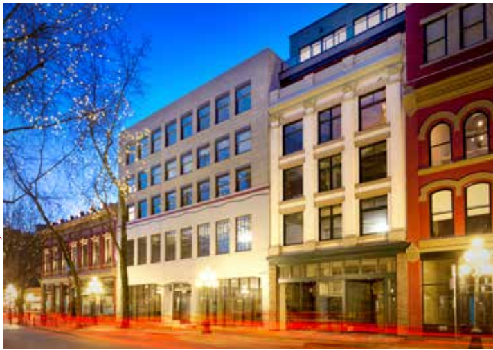
Photo : Action Ostry Architects Inc.
