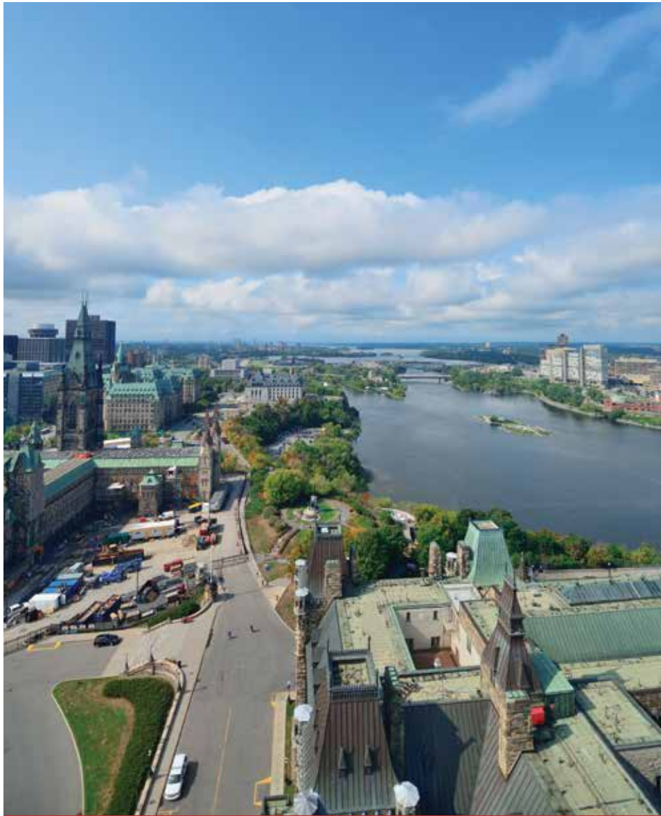
View upriver toward the Chaudière Falls taken from the Peace Tower. Mackenzie Tower and the West Block are visible on the left, with the Supreme Court of Canada in the middle distance.
