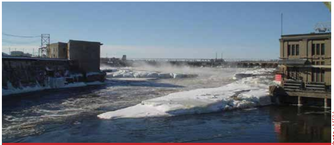
An early spring view of mist rising from the dammed waters of the Chaudière Falls. The first hydroelectric generating station was built in 1912.
