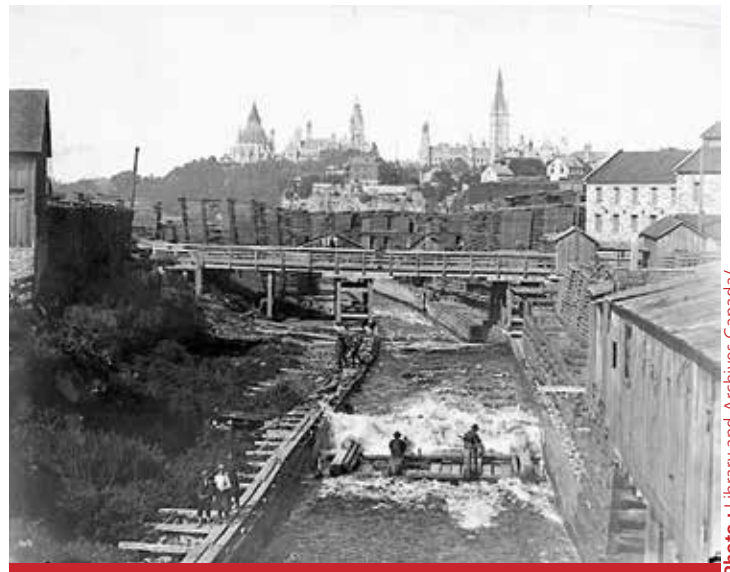
Taken circa 1890, this view of the Chaudière timber slide (water-filled chutes built to carry rafts of squared timber around falls and rapids along the Ottawa River) and some of the millions of board feet of stacked lumber reveals the level of industry at the foot of Parliament Hill.
