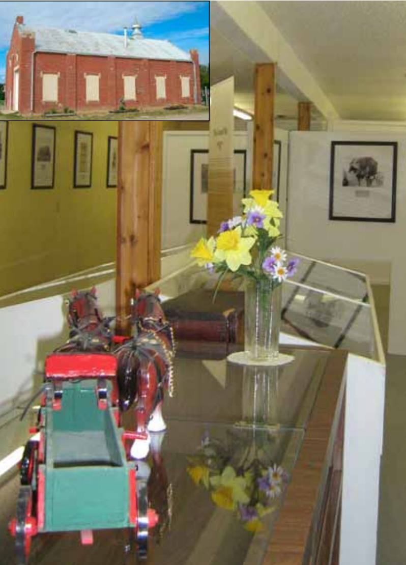
Dating from 1913, the former Melfort power house has been home to the Melfort and District Museum since 1973.
