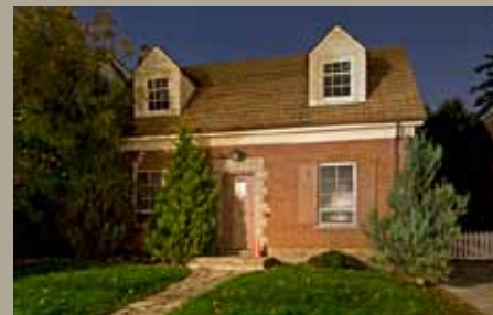
Substation House 640 Millwood Road
