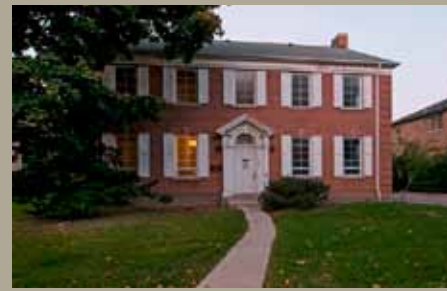
Substation House 555 Spadina Road
