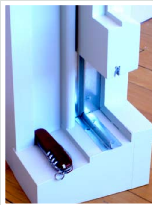
This mock up shows a type of weather stripping where sheet metal fins fit into sheet metal lined kerfs in the sash.
