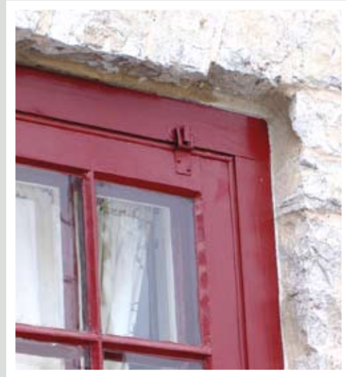
Traditional top hooks or 'storm hangers' are still commercially available and make installation much easier.
