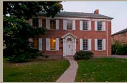
Substation House 555 Spadina Road
