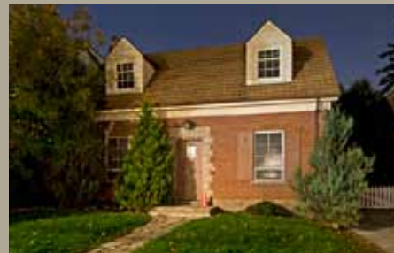
Substation House 640 Millwood Road
