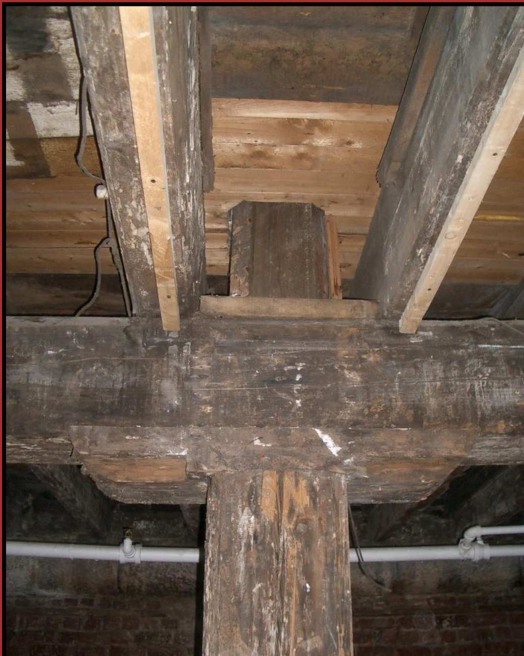
Heavy timber construction
