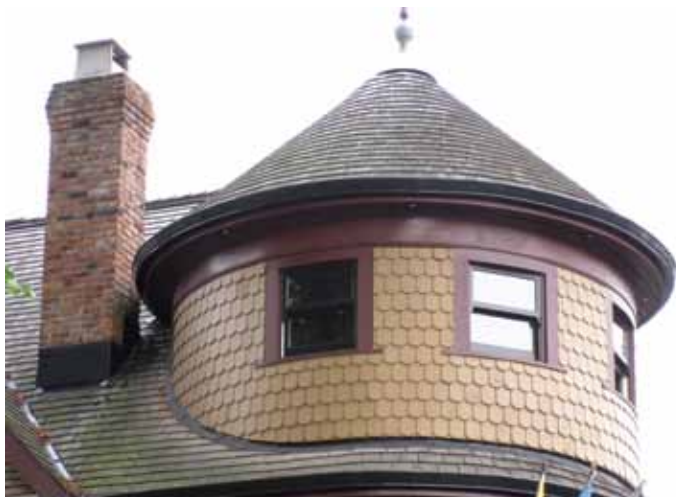
Example of overlapping shingle installation—both a practical and attractive covering.
