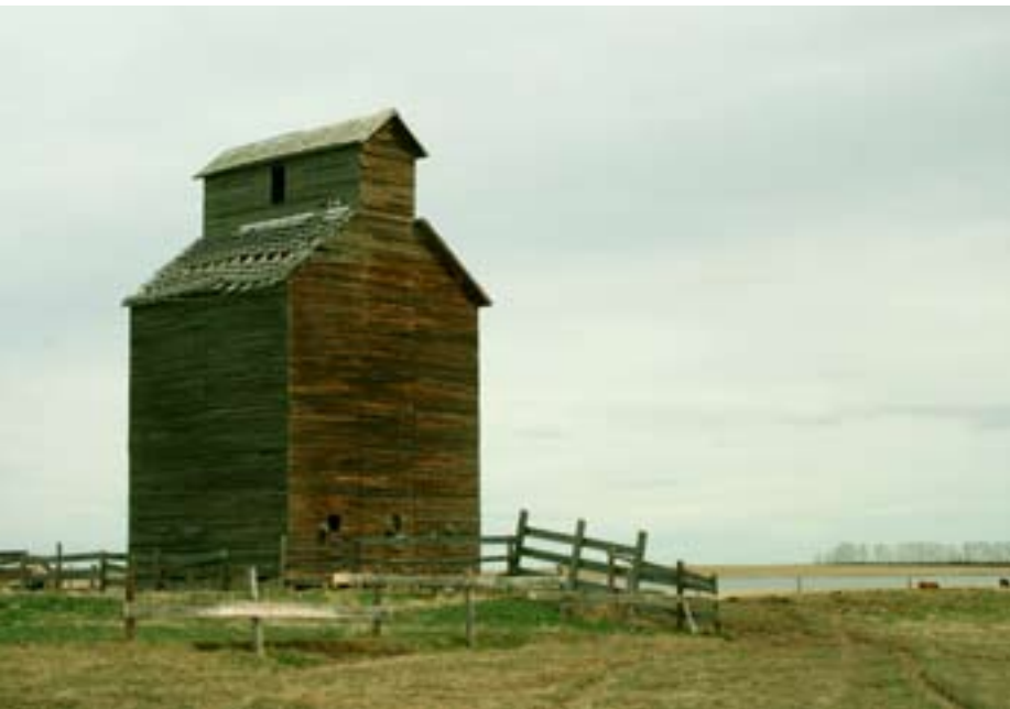
Clear Lake grain elevator, Alberta
