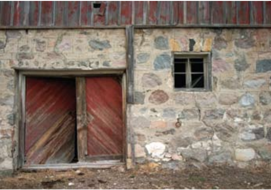
Doune Lodge barn (1903) near Arcola still survives.
