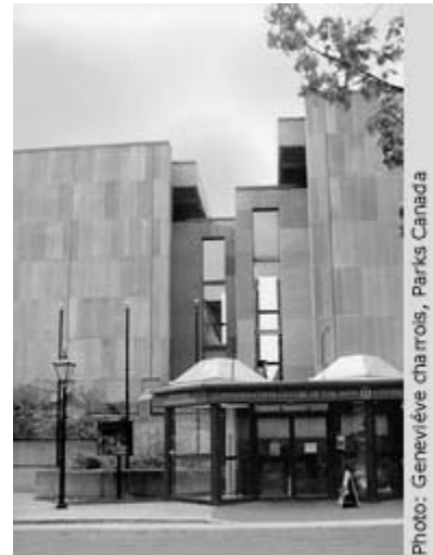
Monolithic forms make up the Brutalist architecture of the Confederation Centre of the Arts.
