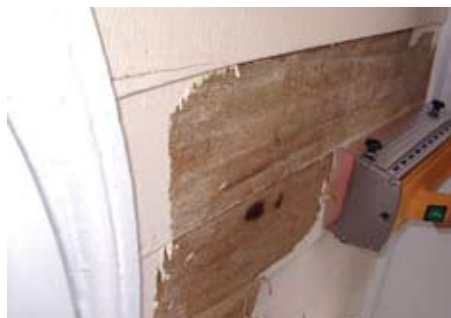
Removing accumulated paint using infrared system and hand scraping technique.
