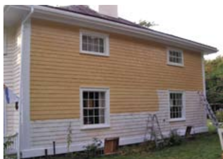
The side wall primed with its first top coat nearly finished.
