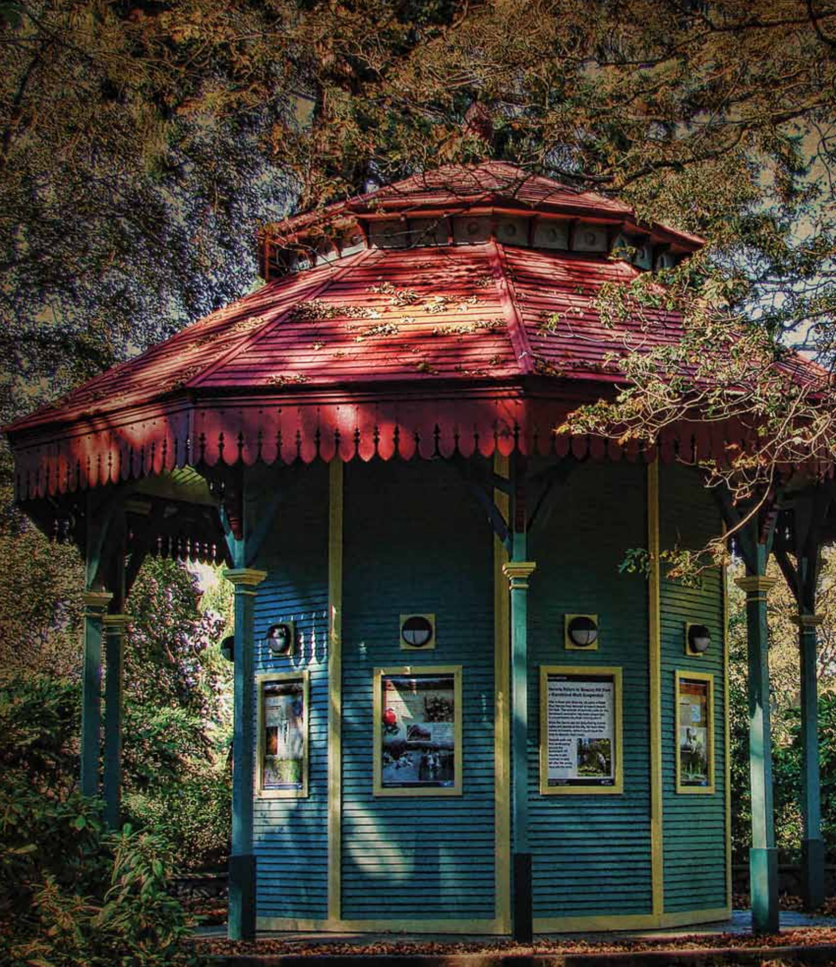
Dating from 1888, the picturesque bandstand is the oldest structure in Victoria's Beacon Hill Park. It was carefully repaired and restored to its original colours in 2010 for use as a new information kiosk.
