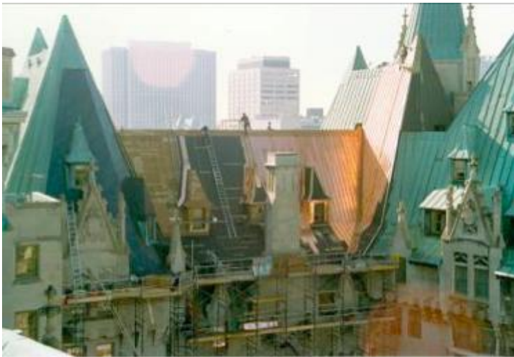
Restoring the Château Laurier roof, Ottawa
